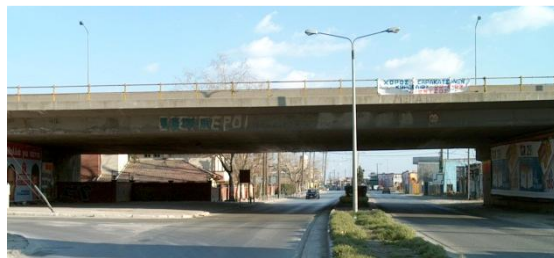
Ring road Interchange K17
