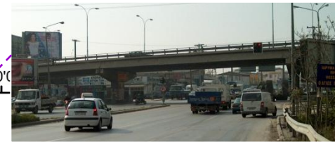
Ring road Interchange K18
